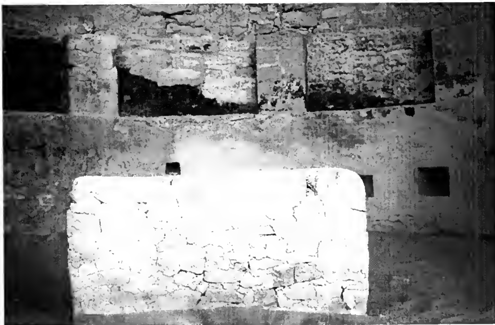
Figure 13. Kiva Q, east wall, deflector.
